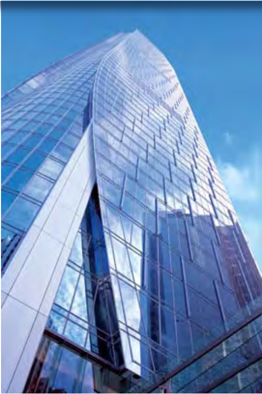
One Island East exterior wall
