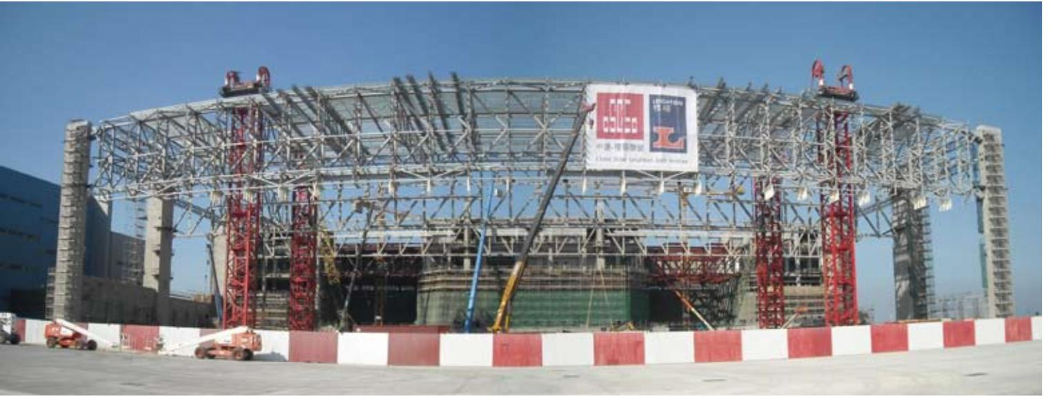
completion will have a clear span in excess of 150 metres. It is steel truss weighing over 2,000 tonnes and will be constructed at ground level and lifted into final position with strand jacks. The project also involves the installation of a foam deluge system and computer controlled access scaffold that automatically encloses the aircraft and provides maintenance access to the entire plane.
