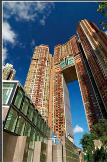
MTRC - Kowloon Station Development
