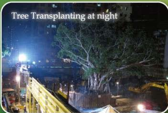
Transplanting of tree with total weight 200 tons
