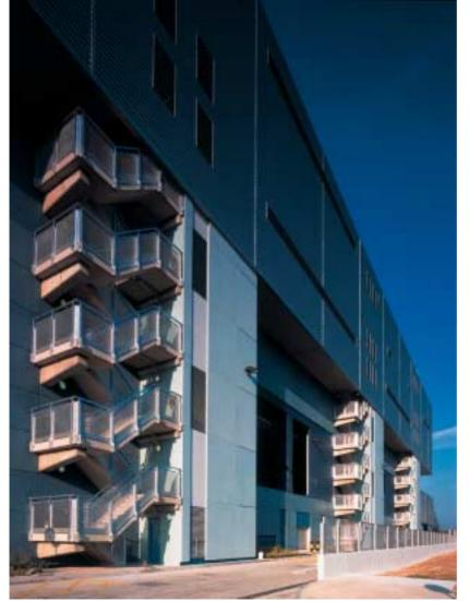
The Tradeport Logistics Centre project followed green construction principles with precast concrete beams, precast staircases and lost form wall panels all greatly reducing the need for traditional timber formwork and allowing a quicker construction program. All floor slabs inside the building were made from pre-constructed T-beams barged in from China.
