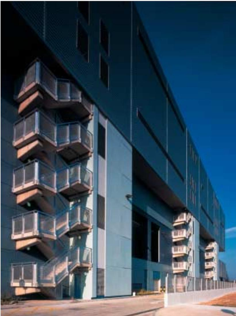
The Tradeport Logistics Centre project followed green construction principles with precast concrete beams, precast staircases and lost form wall panels all greatly reducing the need for traditional timber formwork and allowing a quicker construction program. All floor slabs inside the building were made from pre-constructed T-beams barged in from China.
