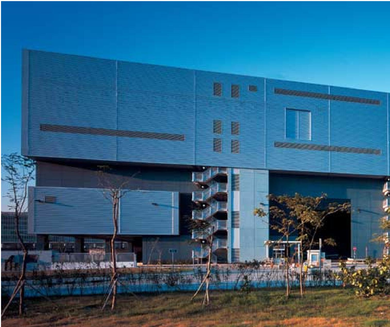
the repeated use of profiled metal cladding at the lower mezzanine floors expresses the movement of the 'containers' sliding towards east and west.
