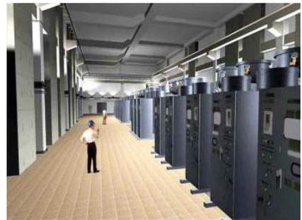
132kV switchgear room with integrated electrical equipment and building services
