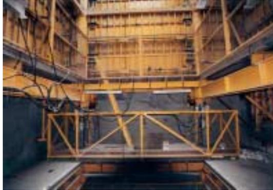
Photo 18: The shutter panels, girder support and hydraulic jack arrangement of the climb form, as seen from inside one of the core shafts
