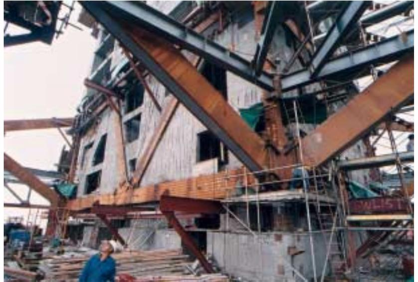
Photo 30: Installation of the outrigger system at 32/F — anchor frame being installed onto the core wall recess. The frame was encased in reinforced concrete at a later stage, after completion of the floor system
