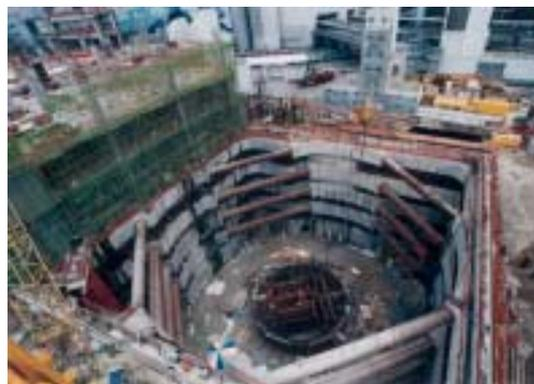
Photo 54: Ground support with waling beams and a corner bracing arrangement to facilitate excavation to form the 32 m deep cofferdam pit
