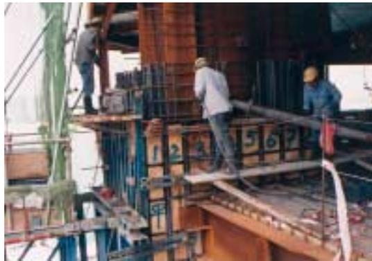
Photo 21: Concreting to the composite mega-column
