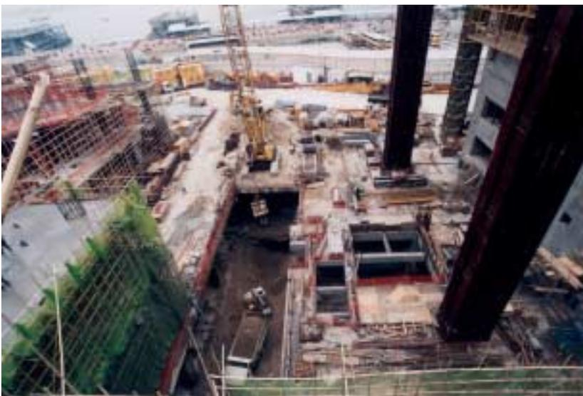
Photo 40: One of the openings provisioned on the ground slab for mucking-out during the basement excavation process
