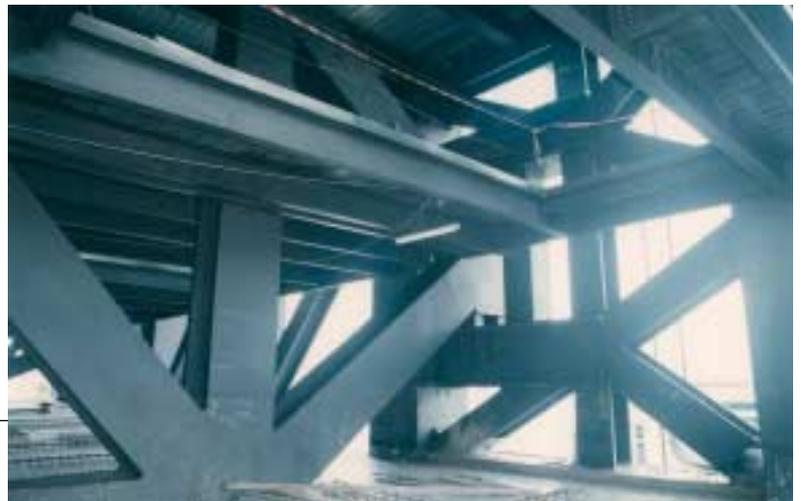
Photo 37: Close up of the outrigger/belt truss joining arrangement as employed at Cheung Kong Center, bearing similarities in design to the Two IFC arrangement
