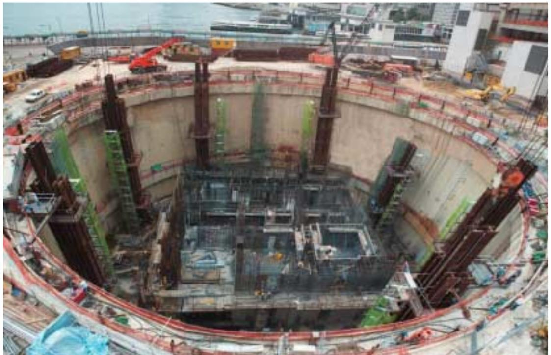
Photo 7: A view into the cofferdam with the core wall and mega-columns in position close to ground level
