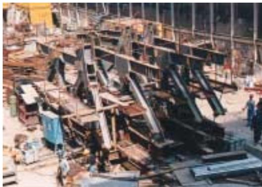
Photo 58: Heavy steel components waiting on the ground before hoisting to work spots at high levels of the tower
