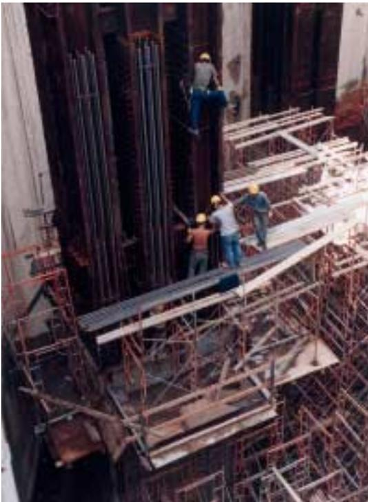
Photo 12: Fixing steel bars (50 mm diameter bars at the base section) around the stanchions of a mega-column before encasing it in concrete
