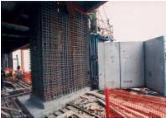
Photo 24a: The climb form in position ready for encasing
