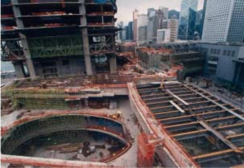
Photo 48: The forming of a 25 m-span oval-shaped atrium with 20 m headroom inside the podium structure
