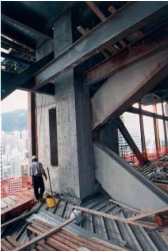
Photo 35: Column joint after the column is encased in reinforced concrete
