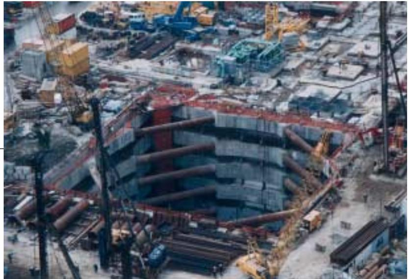
Photo 53: 42 m X 42 m cofferdam formed on the western part of the site for the construction of a vehicular ramp as access into the carpark in the future basement
