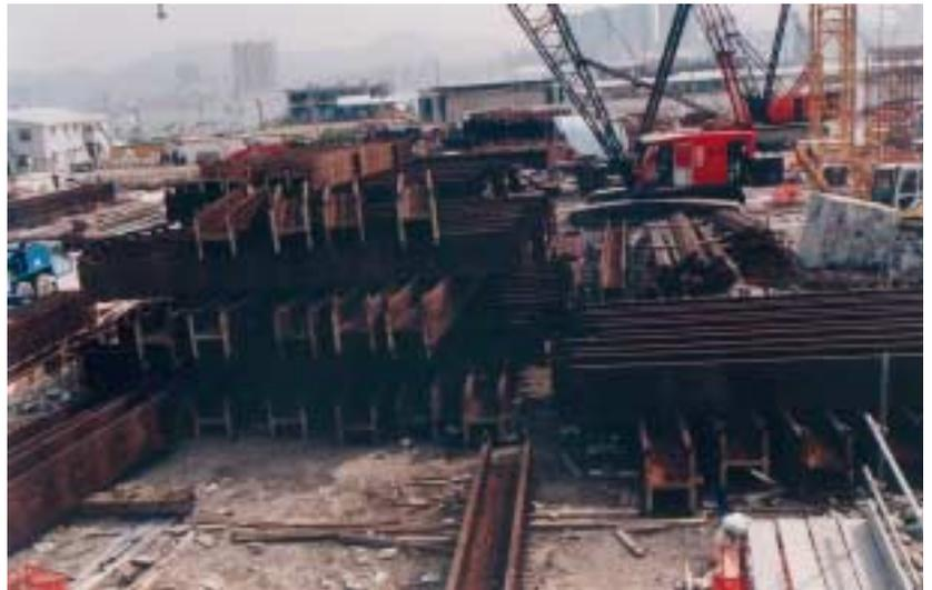
Photo 10: Steel sections stacked on the site for forming the mega-columns
