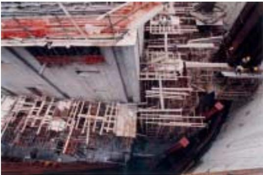
Photo 14: Erection of the first section of climb form at the ground level
