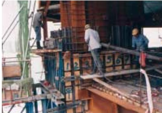
Photo 21: Concreting to the composite mega-column
