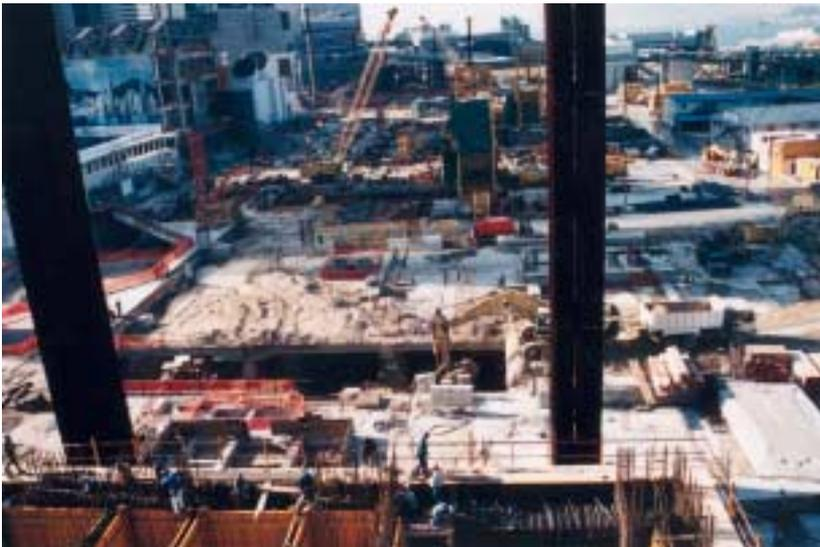
Photo 39: With the ground slab being cast in position, excavation for the basement proceeded in convenient phases. The excavation was initially carried out around the muck-out openings provisioned on the ground slab and gradually extended horizontally and downward in a zigzag manner until basement floors were completed
