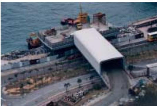
Photo 44: Temporary pier set-up along the seawall outside the site for dumping purposes
