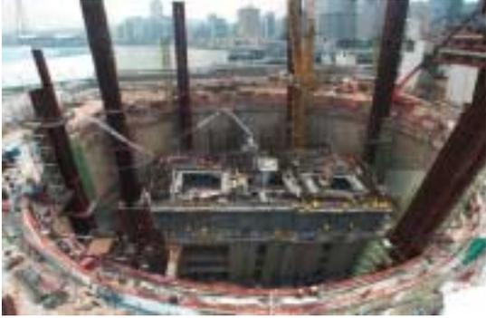
Photo 13a: Close-up view of the formwork system used for the construction of the core wall at the early stage. Another climb form set would be used to replace this when the core wall reached ground level
