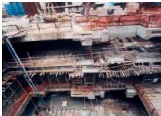
Photo 46: Another section seen through one of the muck-out openings with the double-bit construction arrangement clearly shown
