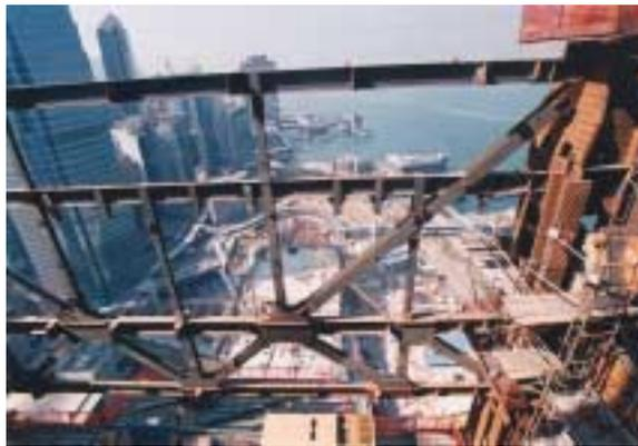
Photo 26: Configuration of the 32/F belt truss before the erection of the floor beams and floor plates
