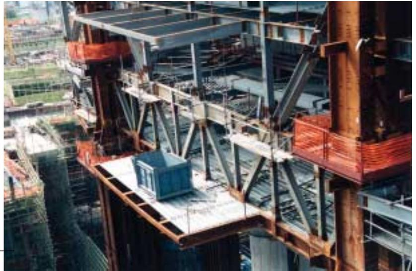
Photo 9: Detail of the south elevation of the transfer truss at 6/F
