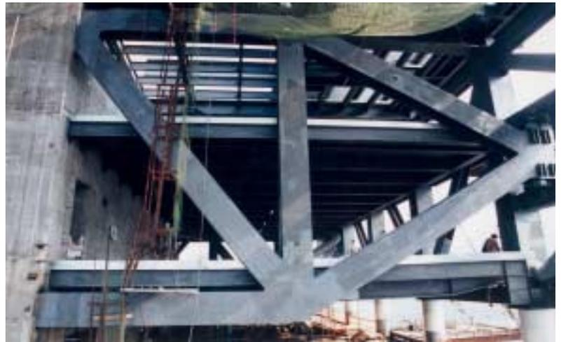
Photo 36: The arrangement of the outrigger system used at Cheung Kong Center (at 59/F)
