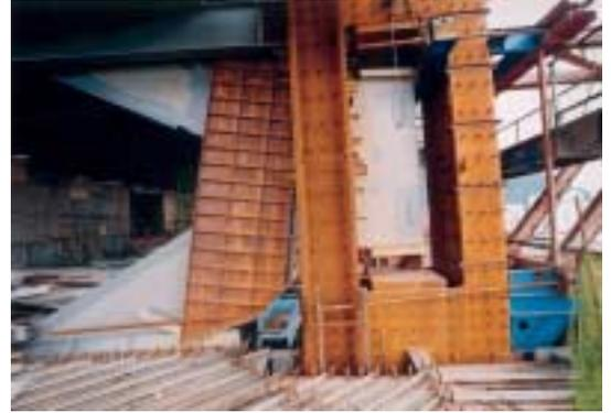
Photo 34: Close-up of the column/outrigger joint with the provision of a slot to control differential shortening
