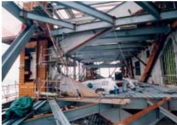
Photo 28: Part-detail of the outrigger/belt truss system at 65/F
