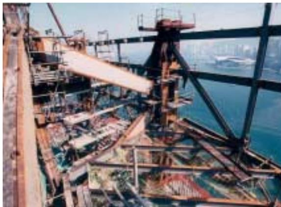
Photo 27: Part-detail of the outrigger/belt truss system at 54/F
