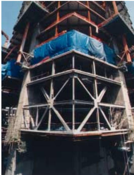
Photo 19: The transfer truss as seen on the 6th floor, supporting two secondary columns at each corner of the building's external frame
