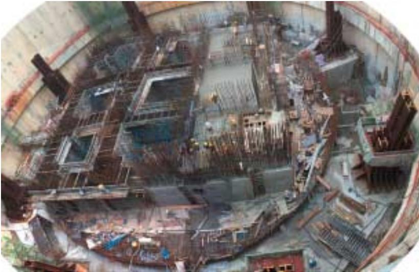
Photo 5: The core wall of the Two IFC tower ascending from the raft at the bottom of the cofferdam. Also note the mega-columns anchored to the plinths by gusset plates
