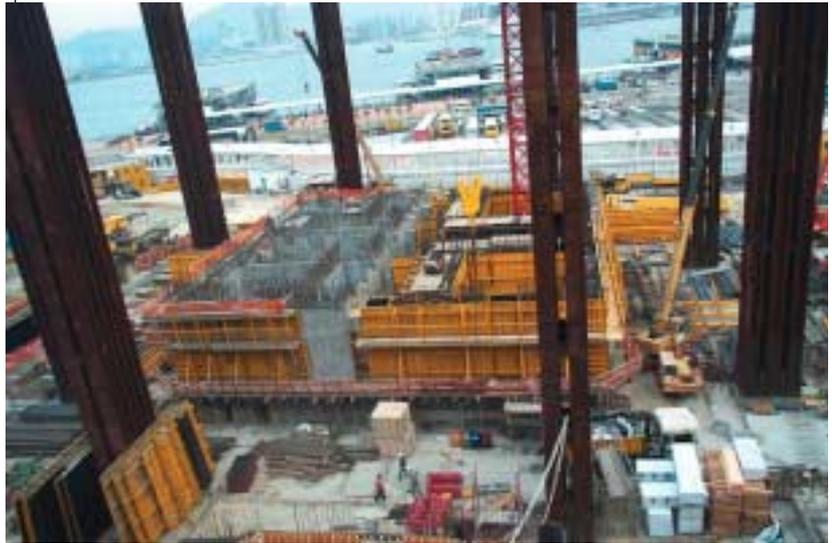
Photo 16: The climb form, composed of two separate climb systems, was used to construct the 780 sq m central core
