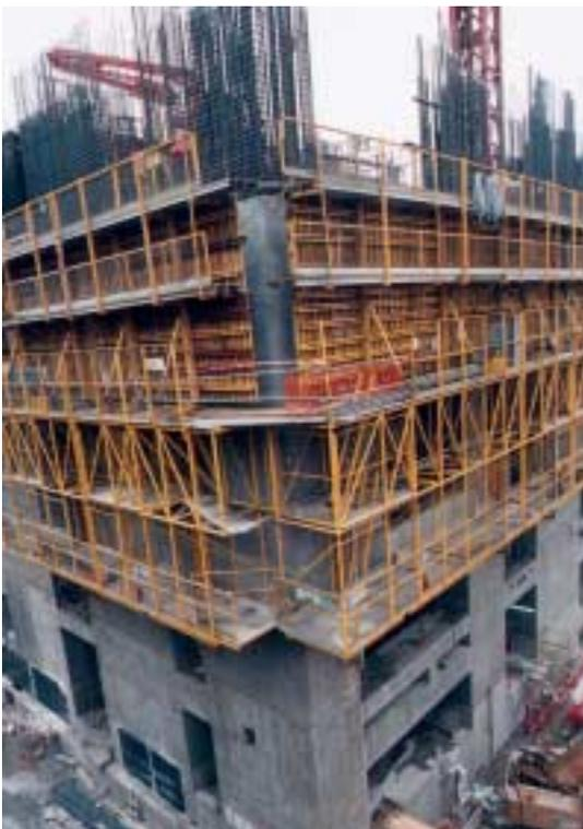
Photo 17: A view of the climb form at a building corner when it was in the released position ready for lifting to the next working level
