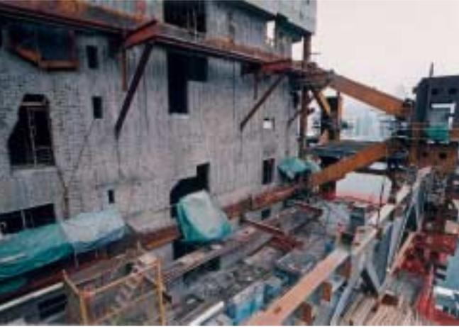
Photo 29: Installation of the outrigger system at 32/F — anchor frame starting to be installed onto recessed positions on the core wall
