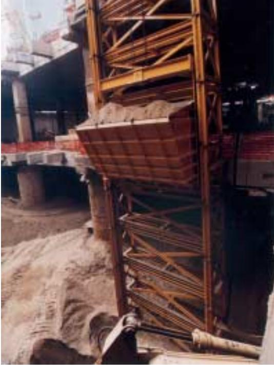
Photo 43: Operation of the spoil removal hoist inside the muck-out opening
