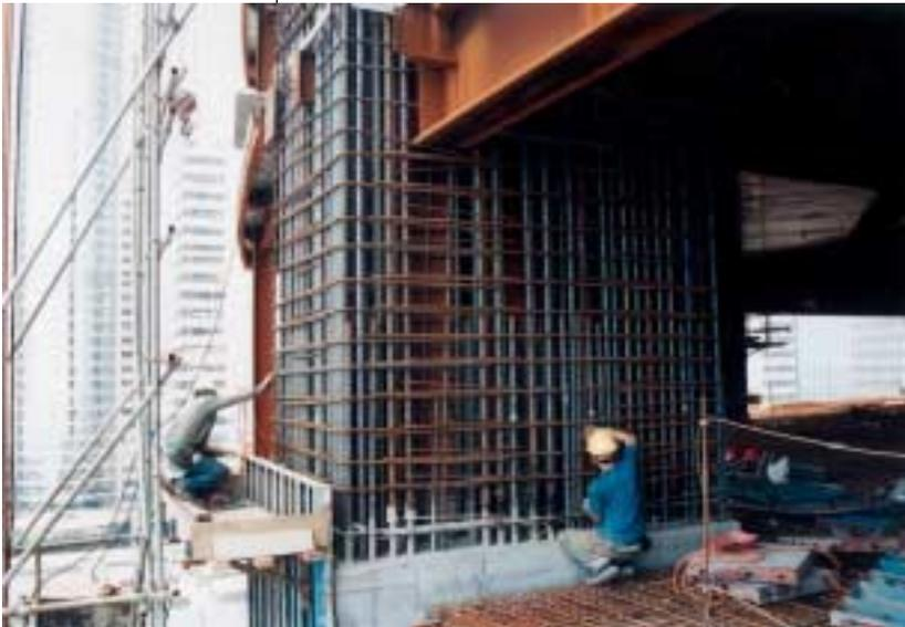
external wall, a deep edge girder spanning up to 24 m is provided to support the floor between the main columns (photo 20).
