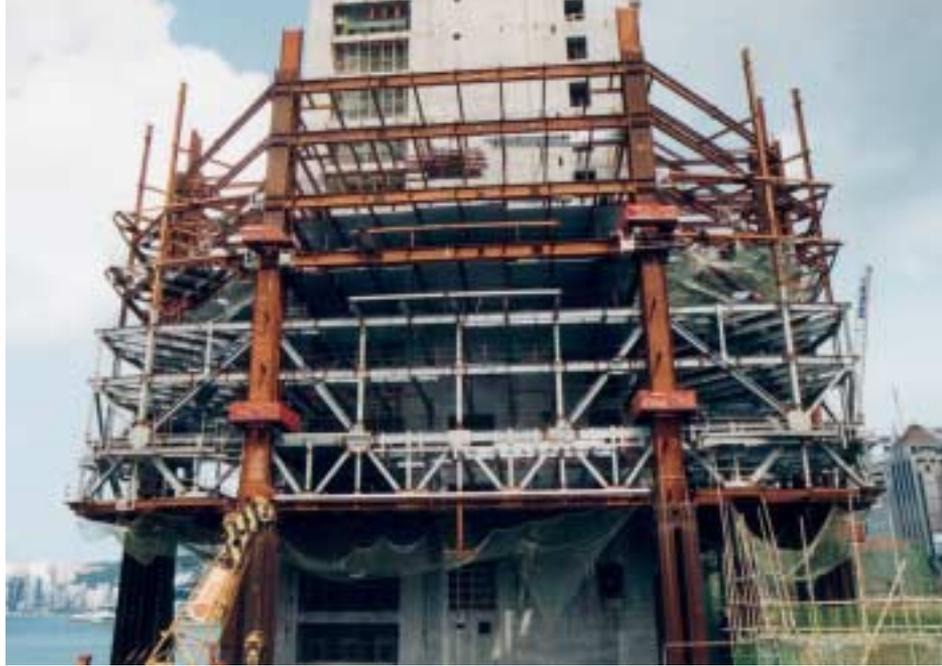
Photo 25: Building elevation showing the basic configuration of the transfer/belt truss at 6/F
