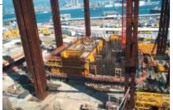
Photo 15: The first section of core wall (western section) being concreted while the erection of the eastern section was in progress
