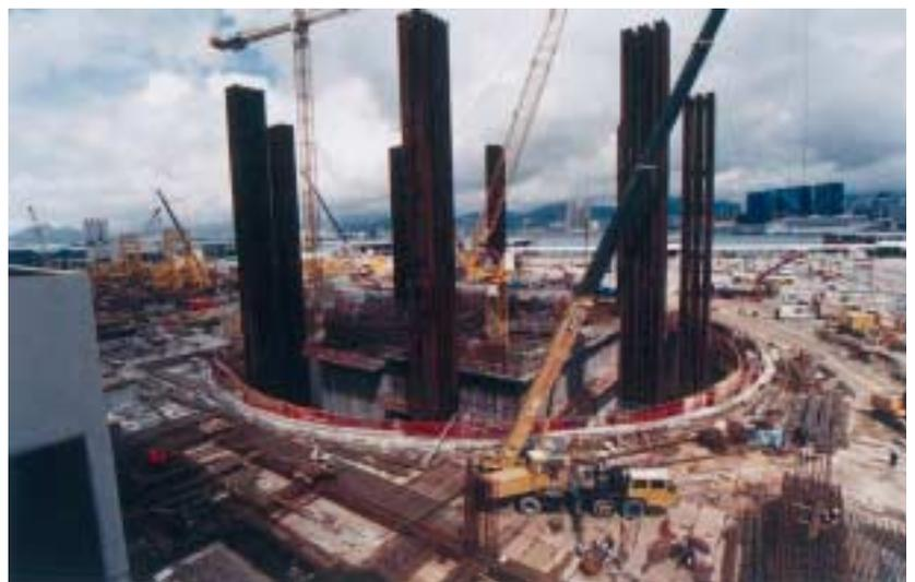
Photo 11: Work stations around the sides of the cofferdam on ground level, forming an important base to serve construction activities inside the cofferdam
