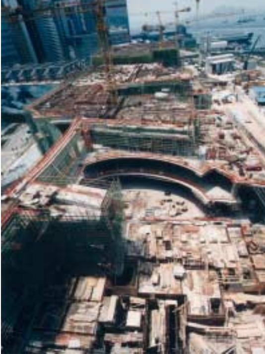
Photo 51b: A close up look at the podium structure which used rather traditional timber formwork in construction
