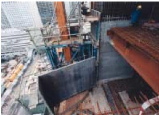
Photo 24b: The climb form in its open mold ready for repositioning to an upper floor
