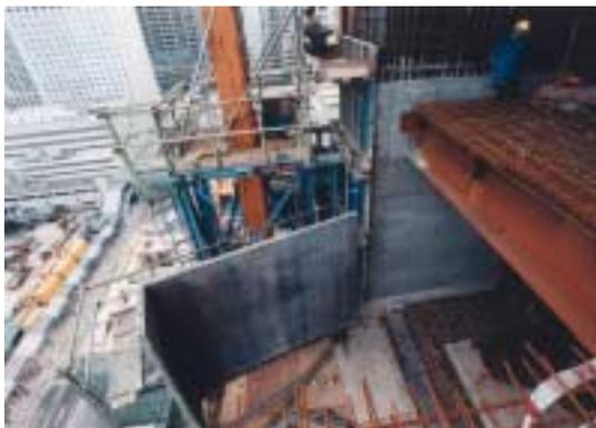
Photo 24b: The climb form in its open mold ready for repositioning to an upper floor
