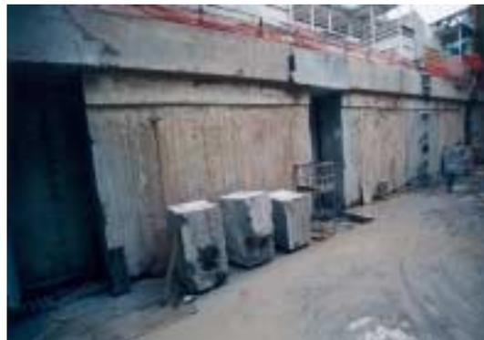
Photo 47: Breaking through into the existing diaphragm wall panels with the saw-cutting method. After removing the wall, the existing MTR Hong Kong Station concourse with the new concourse extension inside the Two IFC basement
