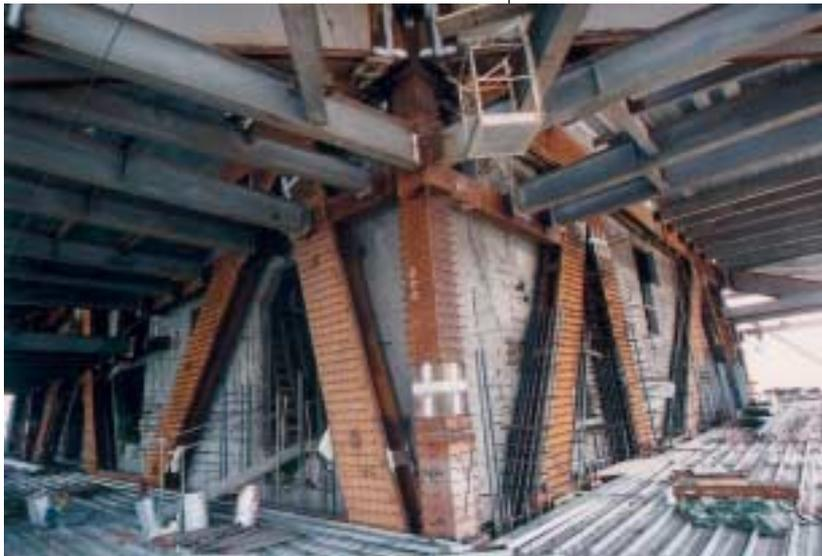
casting (retro-installation) process (photos 29, 30, 31, 32a & 32b), and an external frame in the form of belt truss acting as an external stiffening member and taking up the gravity loads from the corner columns.
